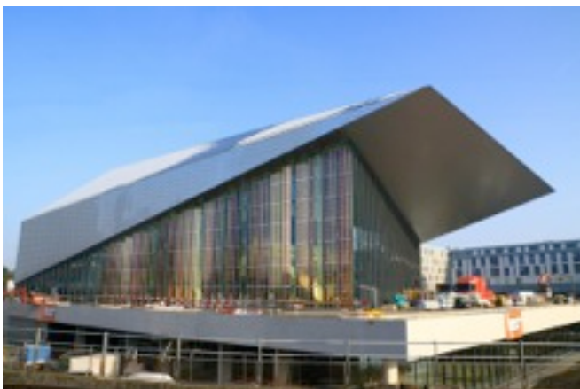
Solaronix' multicolored transparent photovoltaic façade at the SwissTech Convention Center, EPFL, Switzerland.
